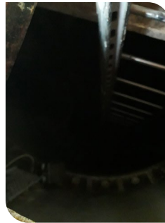
Before: Shaft entrance un-lit
