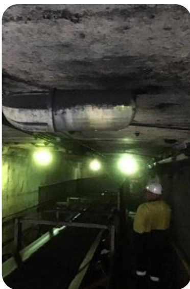
Before: Fluorescent lighting created dark spots along the wash plant conveyor increasing safety risks
