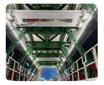
The extra thick copper backbone of the Long-Range LED strip lighting enables continuous run lengths of up to 168 metres. LEARN MORE
